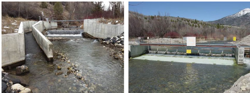
Figure 2. View looking upstream of waterfall-velocity (left) and electric weirs (right) on Burns Creek and Palisades Creek, respectively. The fish trap is located on the left bank at the waterfall-velocity weir and on the right bank at the electric weir.
